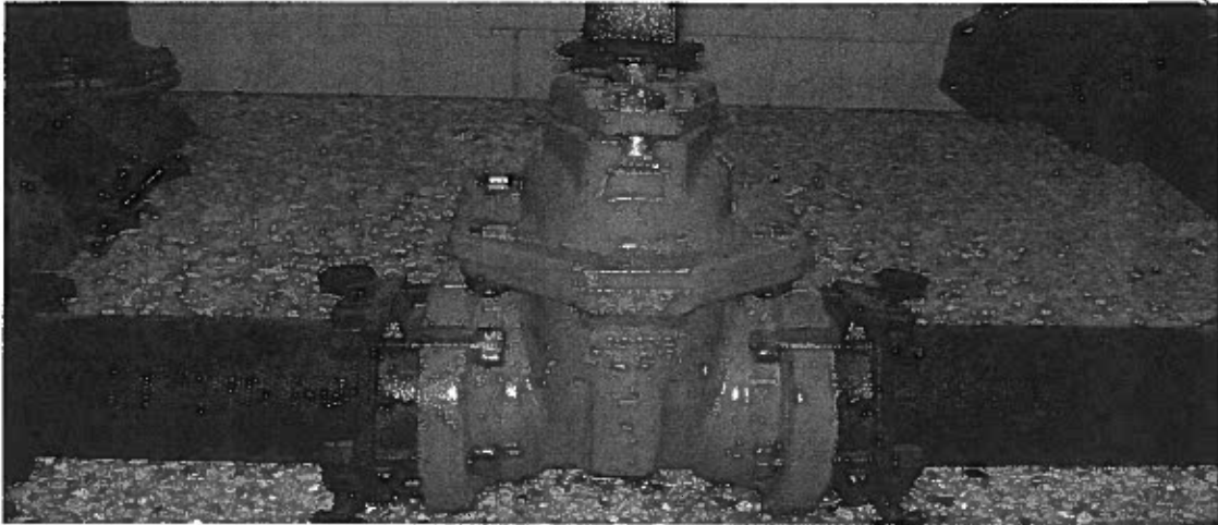
In-line water valve
