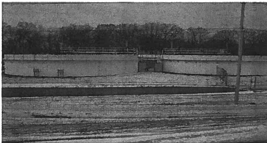
Canoe Brook Circular Clarifiers
