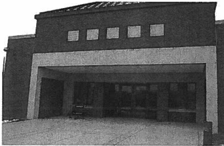
Raritan Millstone Water Treatment Plant
