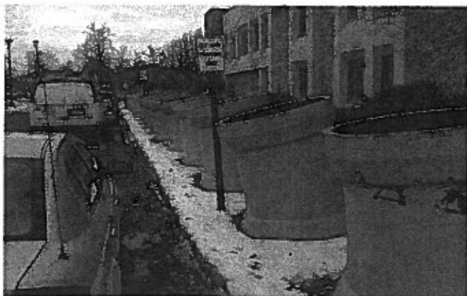
Iron ells in front of plant
